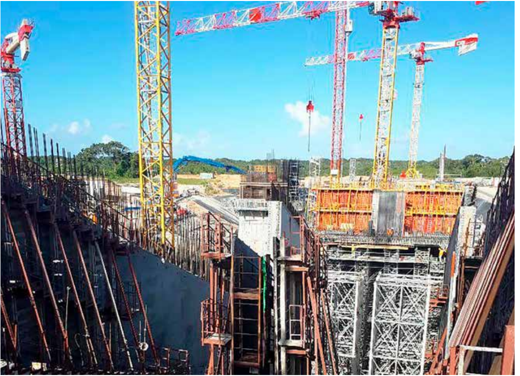
Chantier Ariane 6 © David Fardel
